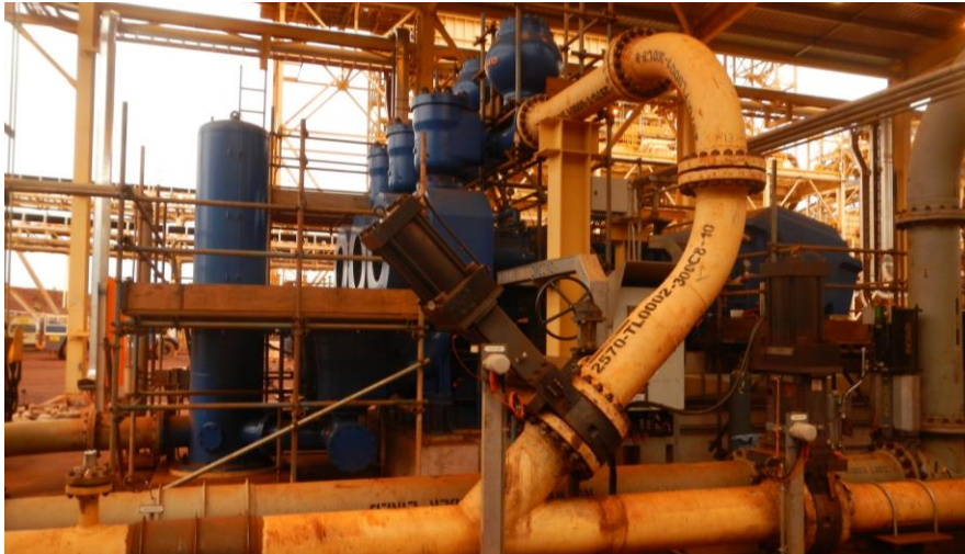
ASME Class 600 slurry knife gate on PD Pump circuit.
