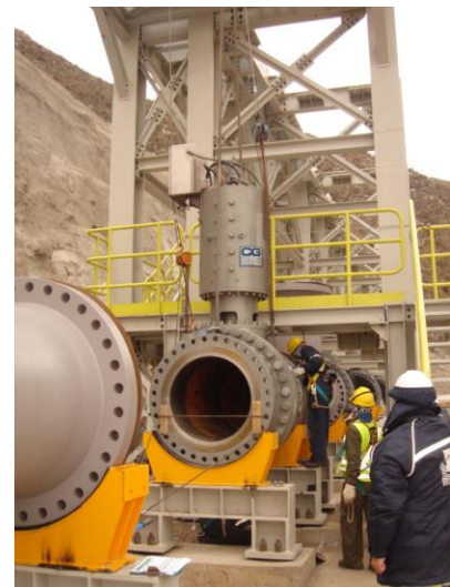
High solids slurry isolation ball valve in a copper concentrate pipeline.
